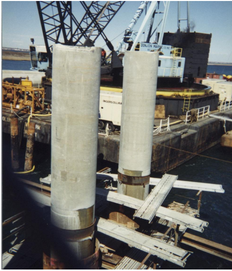
Template for prestressed concrete cylinder pile installation (steel casing has already been removed).
