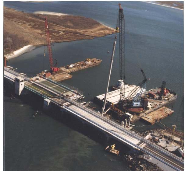
Installation of 160-foot long prestressed concrete cylinder piles adjacent to the existing bascule span, which is on much shorter timber piles.
